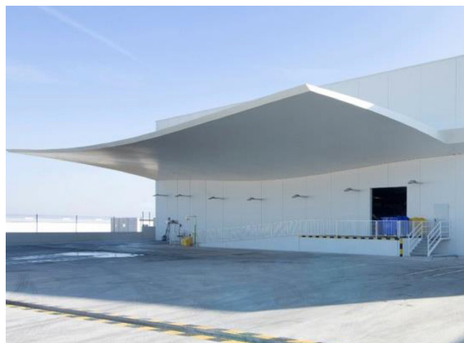
Above: The 340sqm, curved, self-supporting canopy over the loading dock
