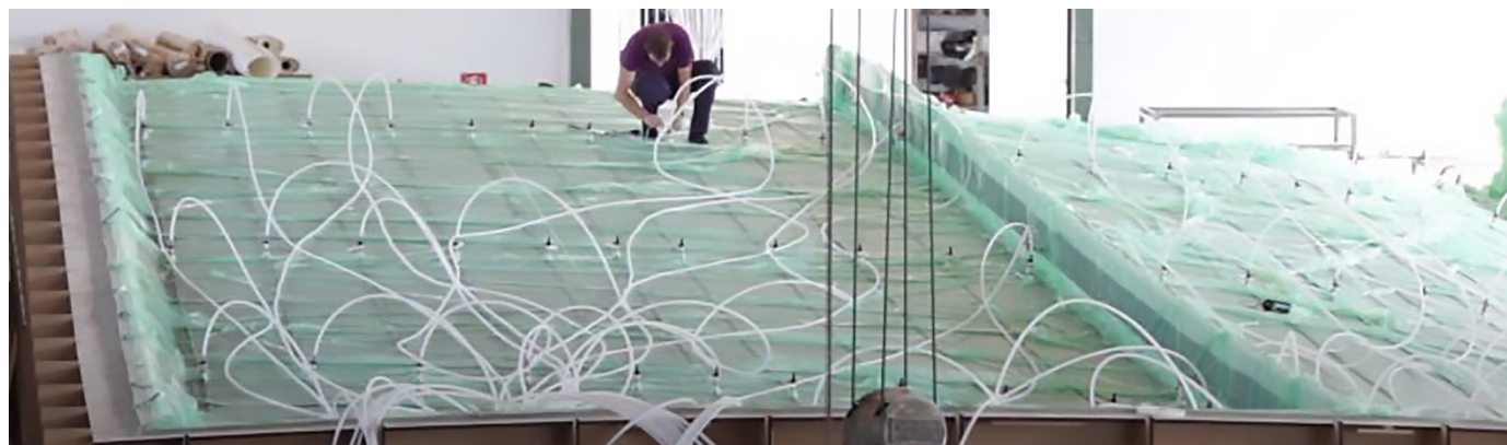
Above: The 340sqm, curved, self-supporting canopy over the loading dock
